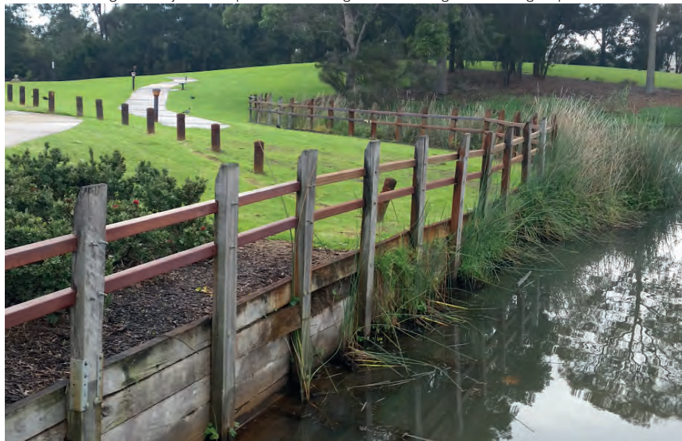
Timber retaining wall adjacent to pedestrian bridge with missing and damaged panels
