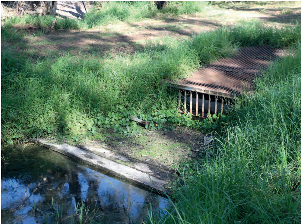
Drainage outlet adjacent to Carslake Grove that takes overflow water to Big Carine Swamp
