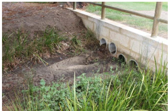
Sediment inflow at Hope St sump
