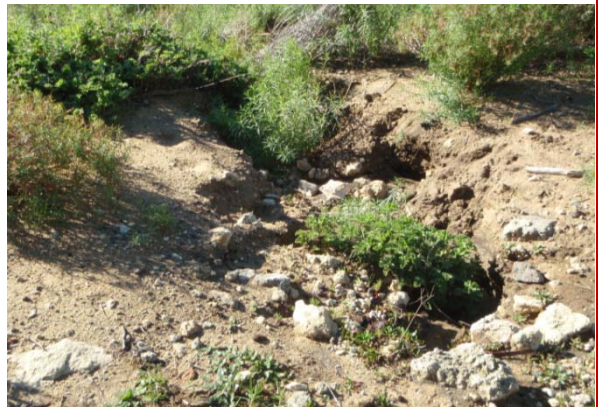
Erosion from water from the Elvire St drain.
