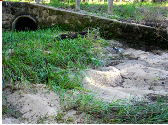
Sediment inflow at Ada St sump, June 18 2012
