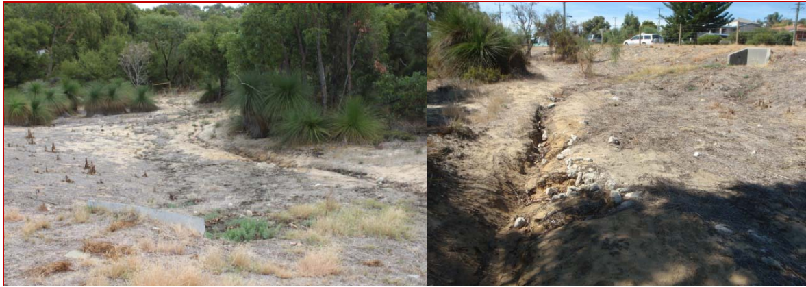
Figure 8: Culvert near Charles Riley Road and Associated Erosion
