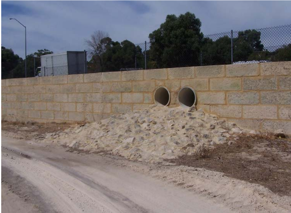
Plate 1: Fauna tunnel linking southern end of Carine ROS under Reid Hwy
